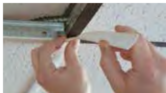
Applying GridMax Over T-bar Suspension Grid System
